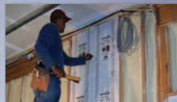
Available in Staple-Tab for wood and Tape-Tab for metal framing
