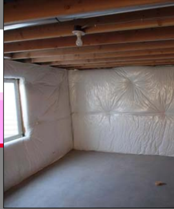
Fiberglass batt w/ vinyl backing
